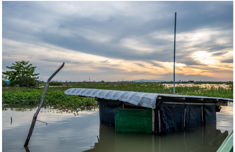
Figure 2: Flooding of the Tonle Sap Lake has rendered this latrine unusable and has exposed the surrounding environment to untreated fecal sludge.
